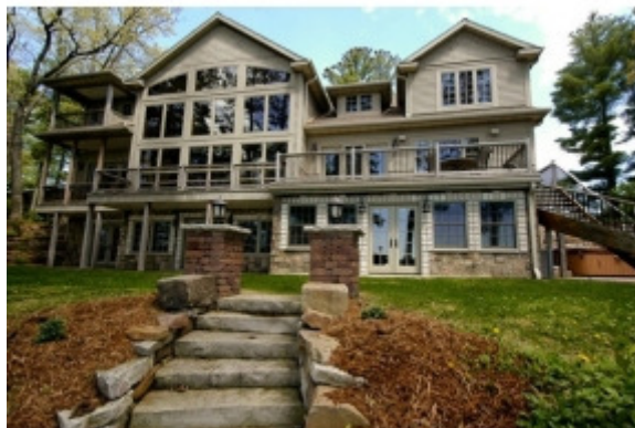
Large Deck Lake Side
