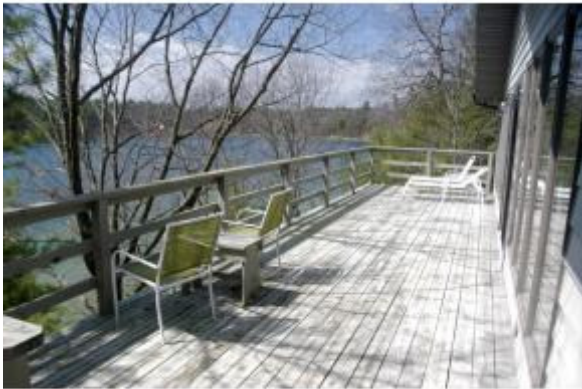
Large Main Floor Deck
